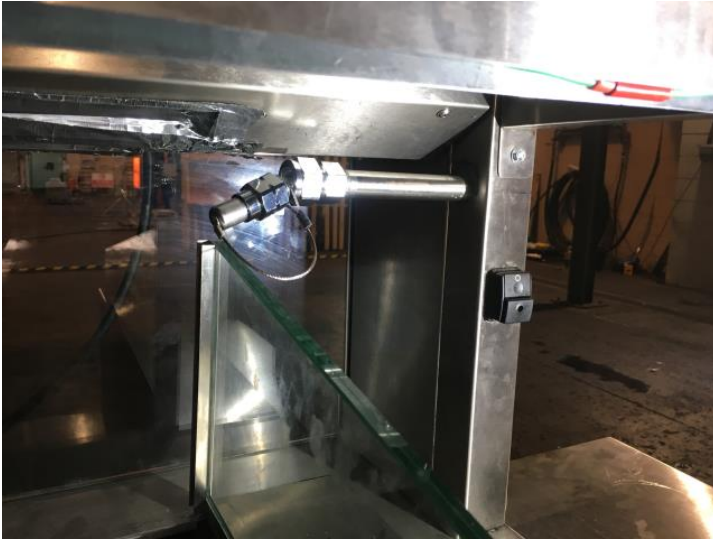
Figure 2 – Nozzle installed over the RHS of the cooking area
