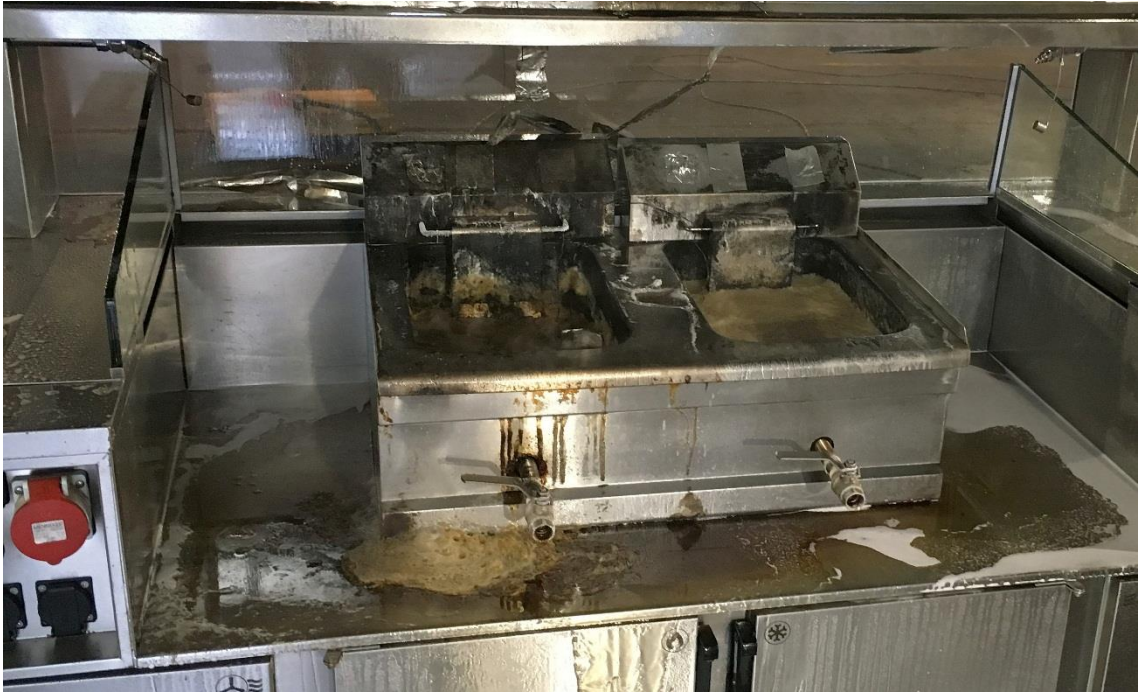
Figure 8 – Test 1, Cooking station post-test
